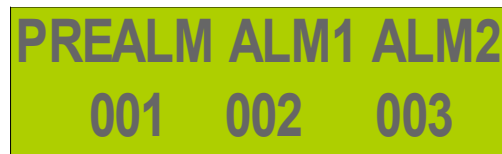
PROGRAMMED ALARM LEVELS
